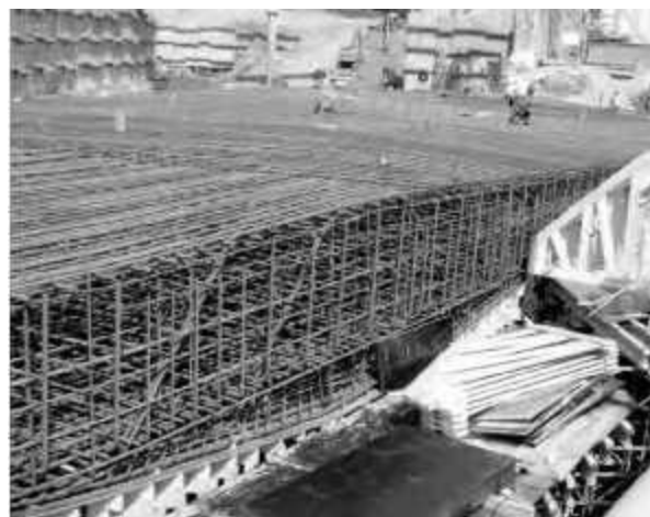
Figure 3.2 – Dalle fortement ferraillées
