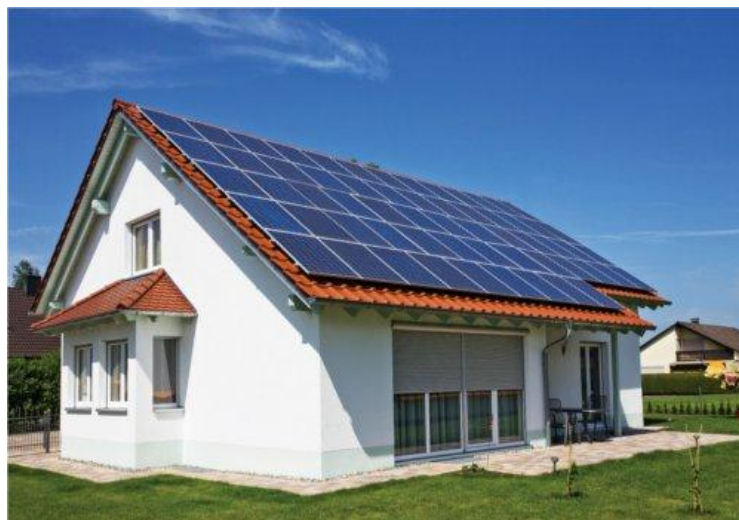
Figure (1-1): Application of Photovoltaic system [5].
