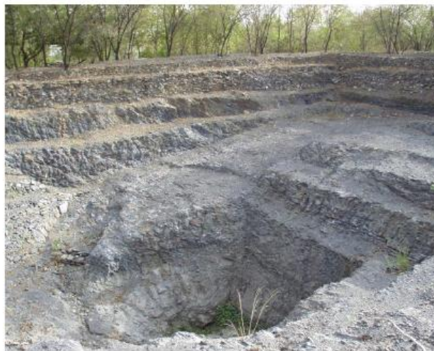
Figure 2.18: Fosse d'infiltration [Gale and al, 2002].
