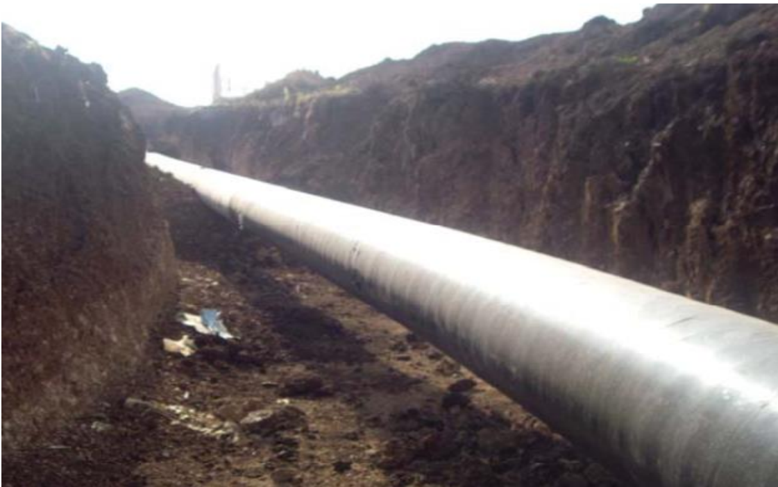
Fig. I.1: Photography of pipeline [2]
