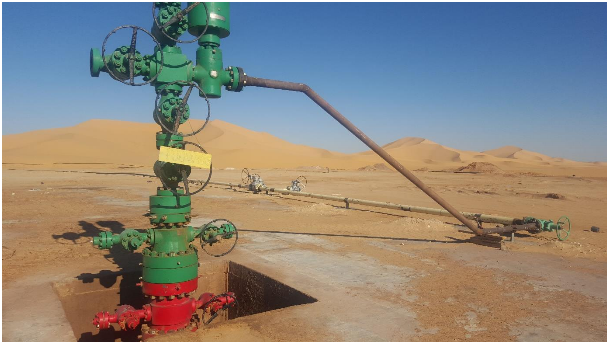
Figure.I.19.Injection point of the corrosion inhibitor
