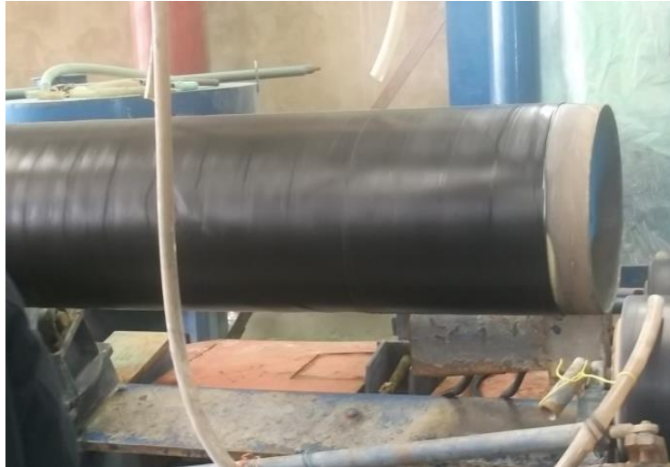
Figure I.16. Coating of outside surface of pipeline with coal tar + epoxy
