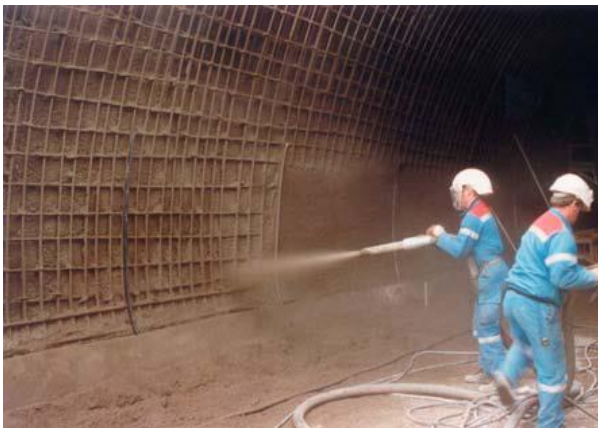
(c)- Projection de béton.
