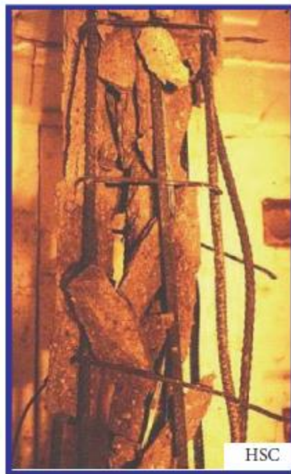
Figure 2. 6 - Relative spalling of high strengths concrete at elevated temperature (Kodur, 2014).
