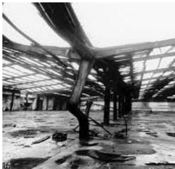
Figure 2. 3 - Buckling problem at high temperature (Wang et al., 2014).
