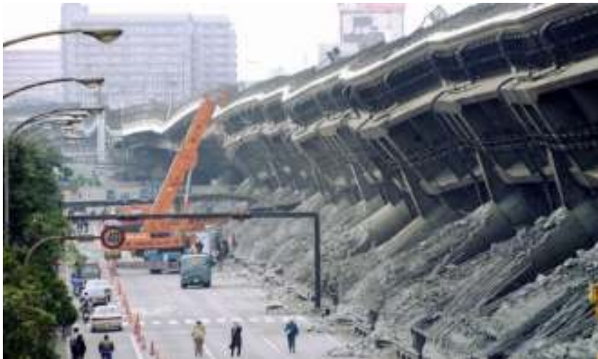
Figure 2.3 Fukae viaduct expressway failure, Kobe, Japan 1995
