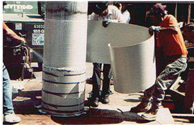
Figure 2.11 RC column confined using prefabricated FRP shells (Kabeyasawa, 2005)
