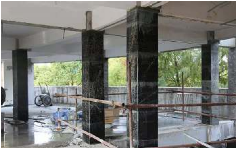
Figure 2.9 Retrofitting of RC columns with CFRP sheets (horseseen.com)
