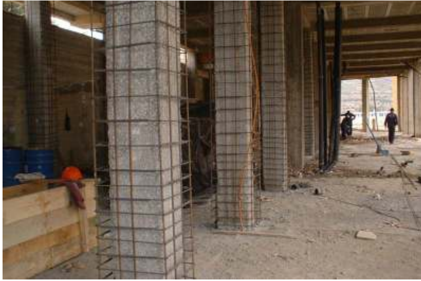
Figure 2.7 Concrete column retrofitted with concrete jackets (Constrofacilitator.com)
