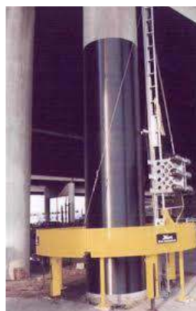
Figure 2.12 Bridge pier retrofitted using FRP automated winding technique (Cozmanciuc et al., 2009)
