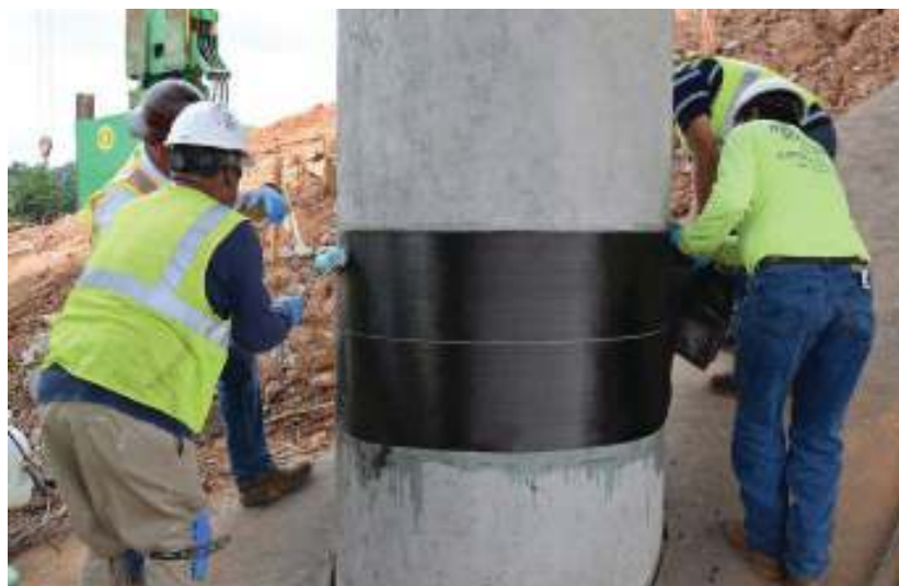
Figure 2.10 Bridge pier confinement using FRP wet-layup technique (informedinfrastructure.com)
