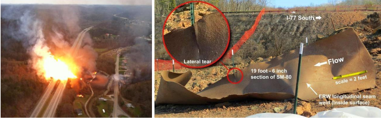
Figure I.3: Incident in Columbian gas transmission natural gas pipeline [13]
