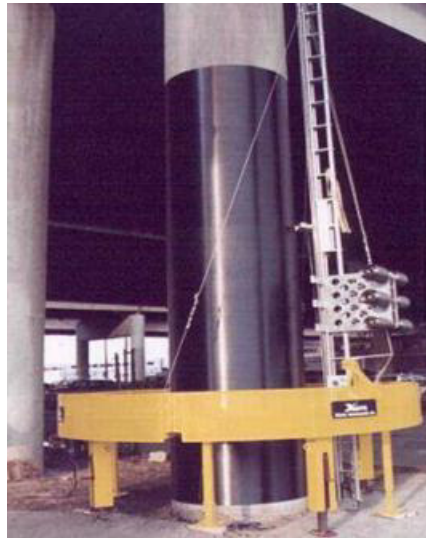
Figure I.23 : L'enroulement filamentaire (Master Builders, Inc. and Structural Preservation Systems 1998, Balaguru et al. 2009).
