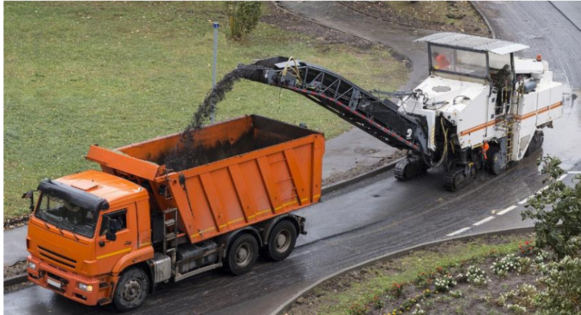
Figure 1. 2. Entretien des routes (fraisage).
