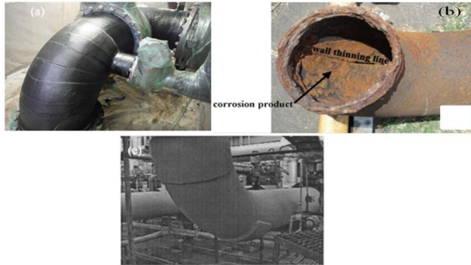
Figure I.11: Different methods of rehabilitation of pipe elbow: composite coating (a), metallic patch (b), and replacement (c) [48, 49].
