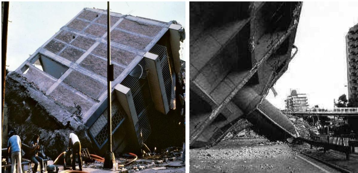
**Fig. 1.2** Settlement of building and foundation failure during Mexico earthquake 1985, [Britannica Editors of Encyclopaedia \(2023\)](#).
