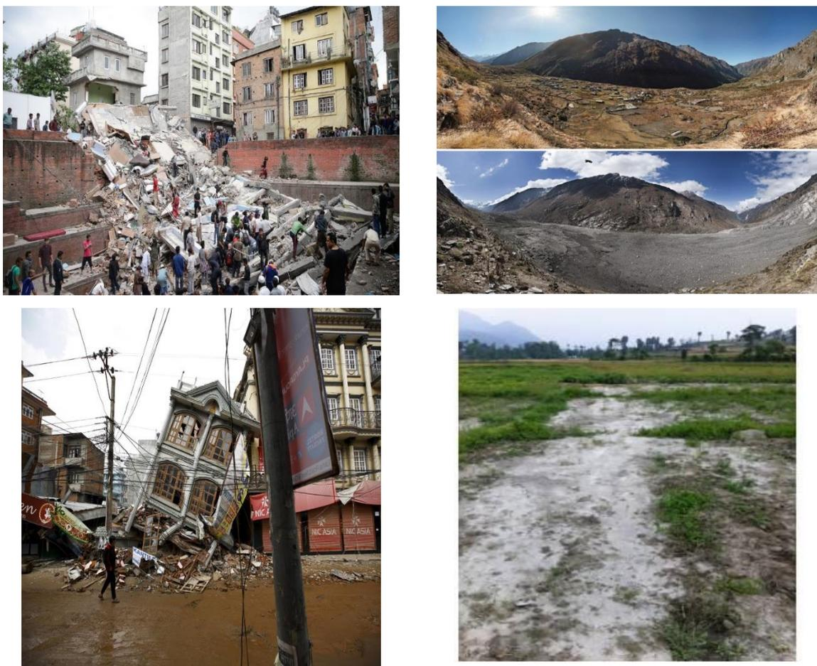
**Fig. 1.8** Building collapse, land sliding, settlement, soil liquefaction during Nepal earthquake 2015, [Taylor \(2016\)](#).
