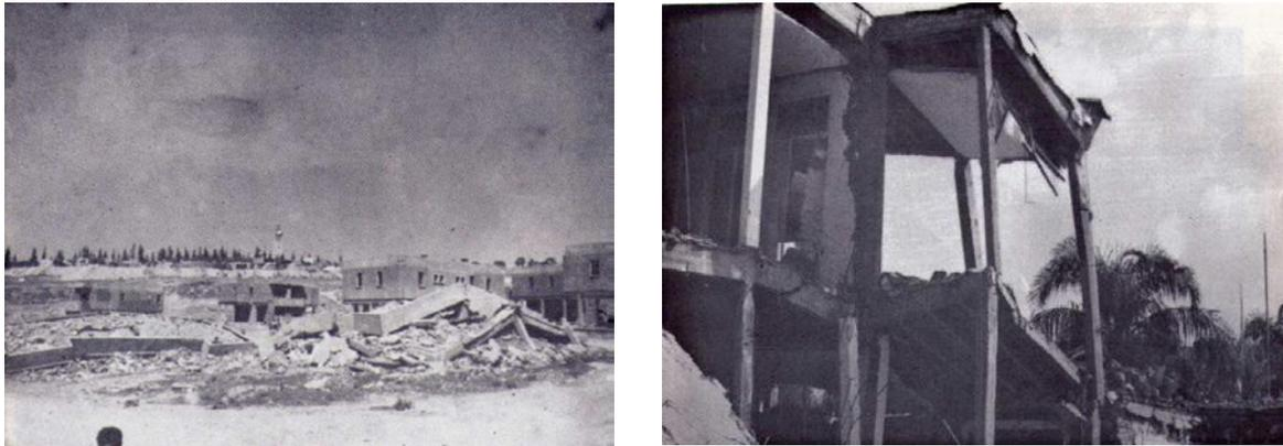
**Fig 1.1** Extent of Building Damage Caused by the El Asnam Earthquake [Ait-Meziane et al. \(2018\)](#).
