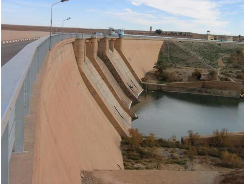
Figure IV.2 : barrage Djorf Torba.
