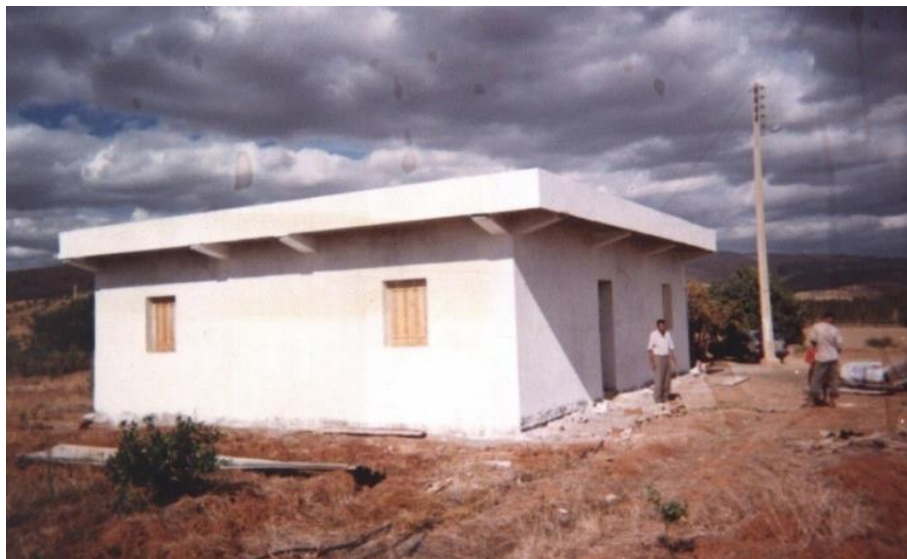
Fig.6.5. Typical rural houses in Chlef with flat roof
