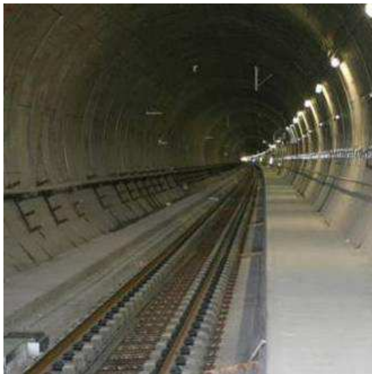
Figure 1.35: Tunnel de Barcelone
