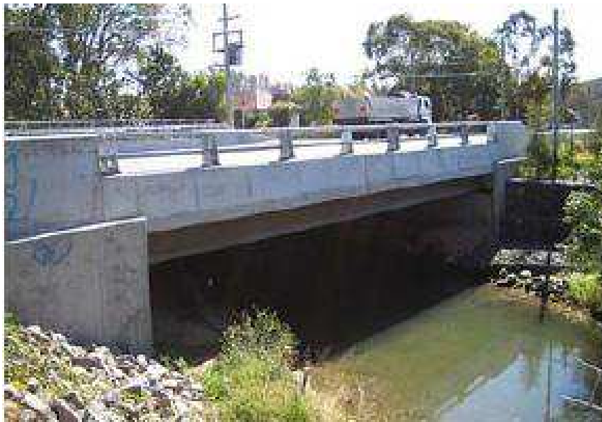
Figure 1.37: Shepherd's Gully Bridge, Australie
