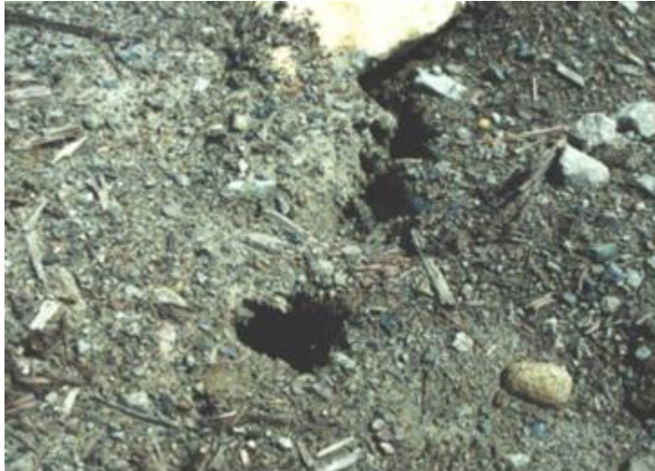
Figure II.5 - Tension crack on road surface
