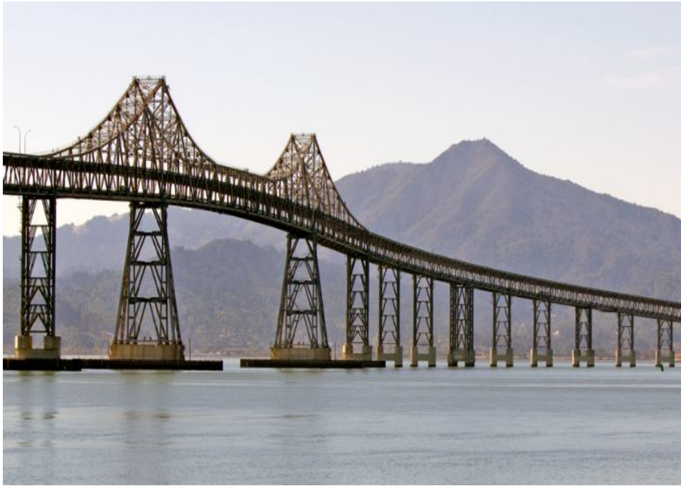
Figure 1-8 : Pont de Richmond-San Rafael, San Francisco [22].
