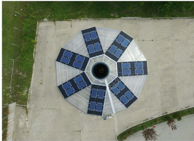
Figure II. 16: Hybrid SCPP Configuration with PV Collector Integration by Eryener and Kuscu [99].
