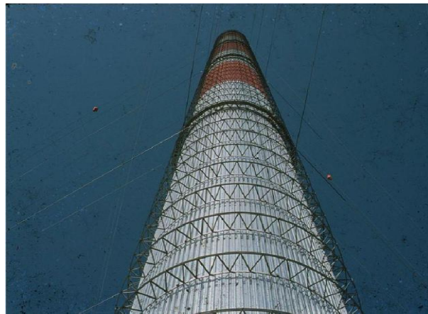
Figure I. 3: The chimney structure of SCPP [11].
