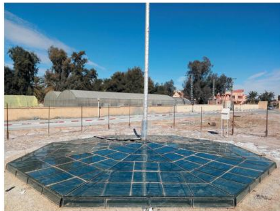
Figure II. 18: Configuration of the Hybrid SCPP with Geothermal Integration by Ouahrani et al [101].
