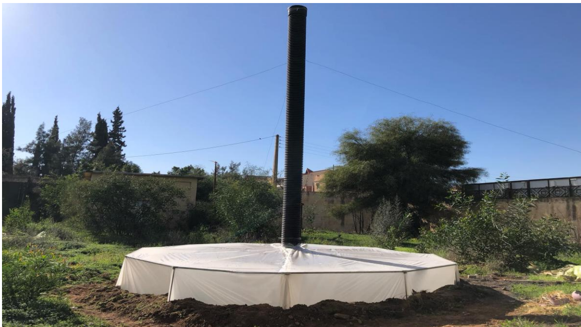
Figure III. 7: Photographic view of the constructed SCPP prototype.
