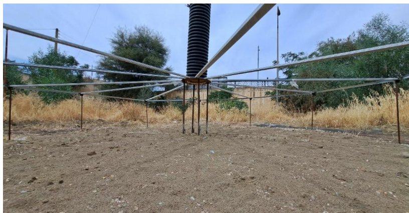
Figure III. 1: Structural frame of the SCPP.
