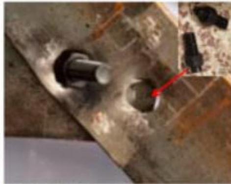
Figure 2-9. Bolt in shear failure mode [138]
