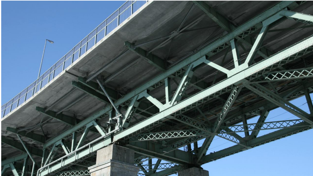
Figure 2-2. Brace connections in the Bridges [137]
