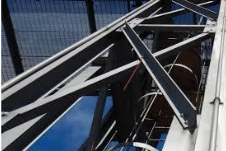
Figure 2-6 Bolted angle steel in braced system [140]
