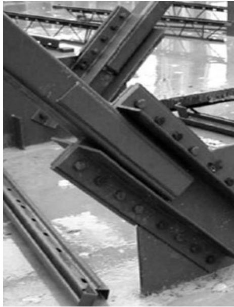
Figure 2-1. Modern seismic brace connection [135]
