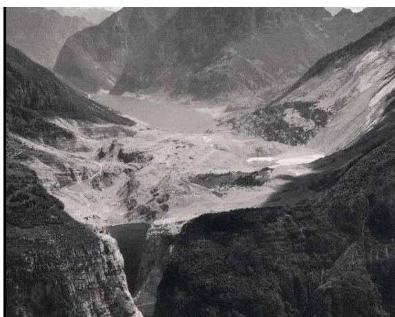
Figure II. 2: Barrage de Vajont (1963) [29]
