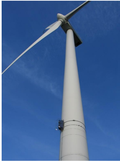
Fig. (1.9): The wind turbine tower.
