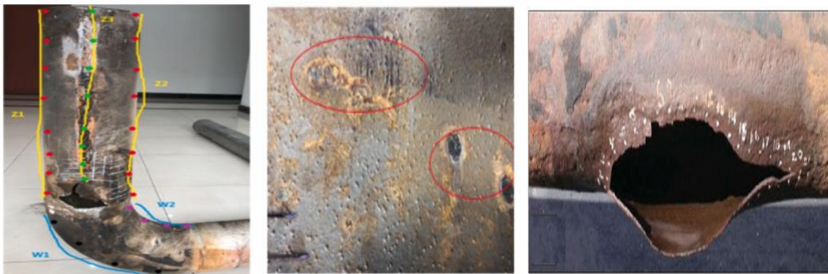
Fig.1.16 Damage of accident pipeline cause interaction steel-flow [30], a) broken pipe, b) morphology insides the rupturefluid [31] and c) fracture due to the SCC, plastic deformation - the local bulging [29].
