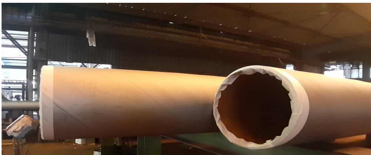
Fig.1.7 Outer pipe stripping
