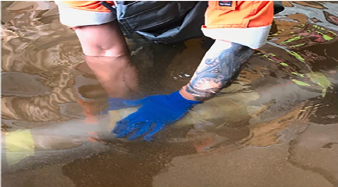
Fig.2. 17 Repairing in water with hybrid glass/carbon layers [175].
