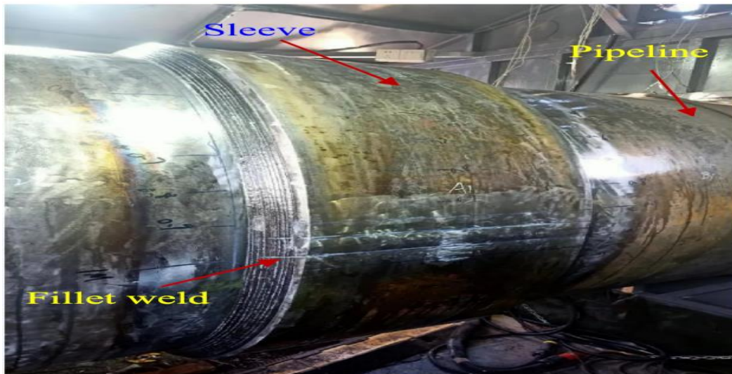
Fig.2.9 Pipeline repair via type B Sleeve [110].
