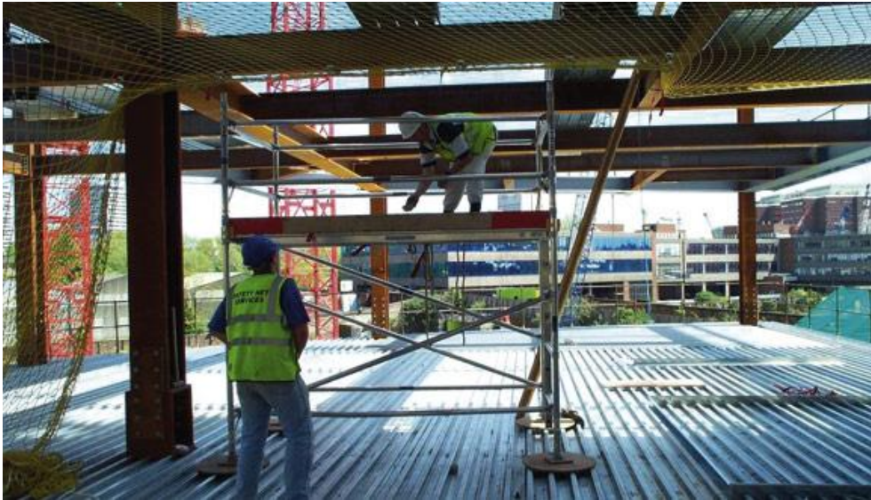
Figure 1.1: Steel deck as a temporary working platform [5].
