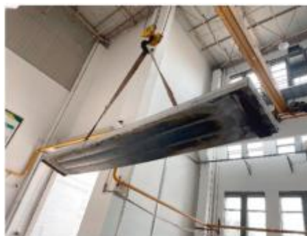
(b) Slab specimen after testing.
