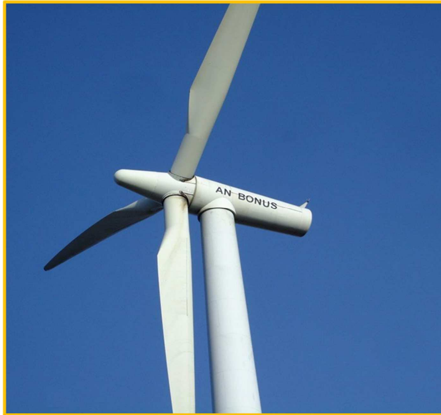
Figure (III-04): The AN Bonus 1000/54 Wind Turbine [18]
