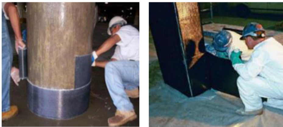
Figure I.33: RC columns Confinement using FRP Wet lay-up process (Chakra 2016).
