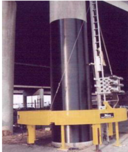
Figure I.36: RC element strengthened using automated winding technique (Master Builders, Inc. and Structural Preservation Systems 1998, Balaguru et al. 2009).
