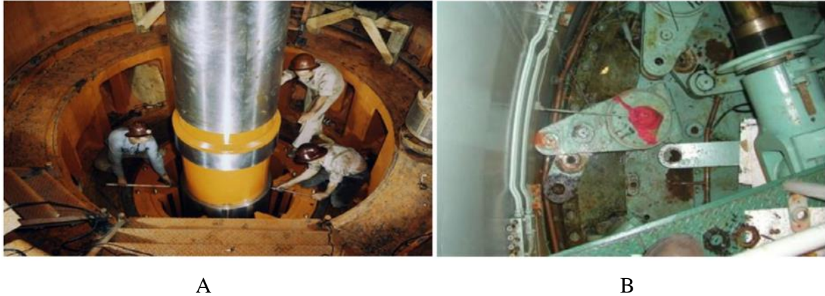
Figure 3: Turbine (A) Misalignment detection [6] and (B) Breakage of Wicket gate linkage [5].
