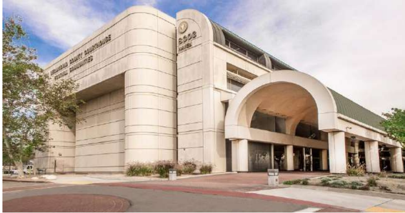
Figure I- 8: Foothill Law & Justice Center (angelescontractor)
