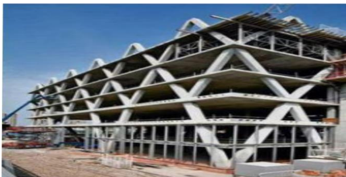
Figure I.11 : Contreventement triangulé[6]
